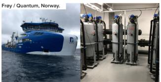
Protection of a reverse osmosis desalination system, used to fill freshwater tanks on live fish transport vessels (salmon farms). A set of AG400 Marine filters at 20  $\mu$ m and 6  $\mu$ m treats the raw seawater, protecting 10  $\mu$ m absolute filters placed before the high-pressure pumps. Total flow rate of 500 m³/h.
