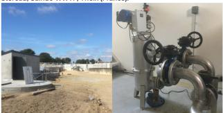
Filtration at the clarifier outlet, before lagooning. AG200 2" 400  $\mu m$  filter.
