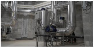
Aquathermie on groundwater for the store's air conditioning. To protect the exchangers, two AS300 DN100, 100  $\mu$ m filters were installed. Insulation was added by the installer.
