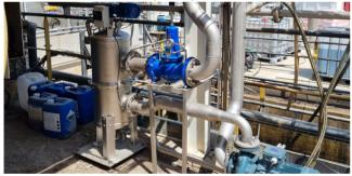
Filter in the treatment of a cooling tower. Bypass filtration: pump + AG300 316L filter (50  $\mu$ m) + VSM pressure maintainer. Flow rate 50  $m^3/h$
