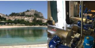
Filtration of a swimming pool. Filtration of the water supply (borehole) (AG400 2  $\mu m)$  and the water in the pool in a closed circuit: three AG400 316L 50  $\mu m$  filters.
