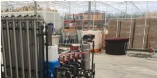
Closed-loop water filtration for greenhouse tomato irrigation. 20  $\mu m$  filtration before UV system.
